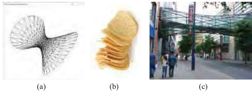
Figure 10.51: (a) Screenshot of hyperboloid1sheet.cpp (b) Edible hyperbolic paraboloids (c) Hyperboloid footbridge over Corporation Street in Manchester in England supported by its rulings (courtesy of Patrick Litherland).
